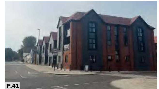
Figure 41: Community Gateway Association - The Watermills development
