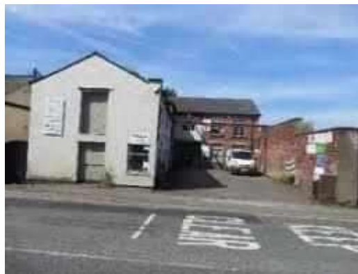
Village Centre post bypass
