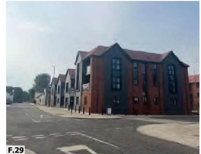
Figure 29: Broughton Village's main intersection between the B5269 and Garstang Road
