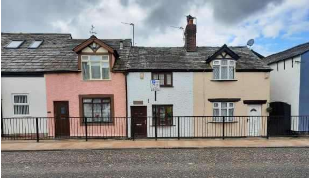
Garstang Road 18 th Century Cottages
